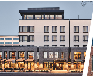
CLAYTON HOTEL Denver, Colorado 63 Rooms
